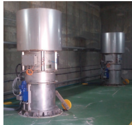
FIGURE 4: Turbogenerator modules.
